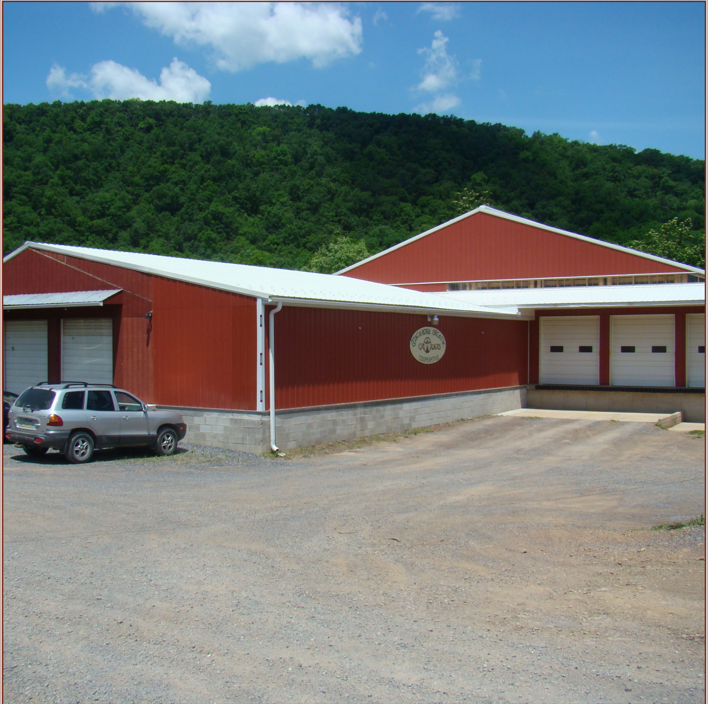
Tuscarora Organic Growers’ current warehouse facility.
