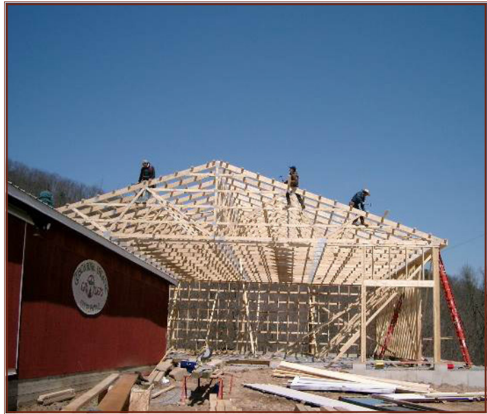
Construction of 2004 addition.
