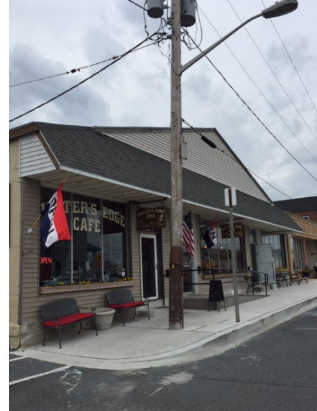
Main street businesses in Crisfield have benefited from sidewalk and street improvements. Photo credit: Renaissance Planning
