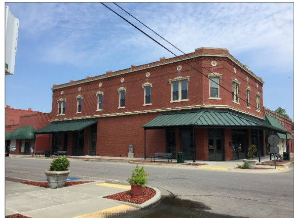
Figure 1 – City Hall building in downtown Lake Village. Image Credit: Renaissance Planning
