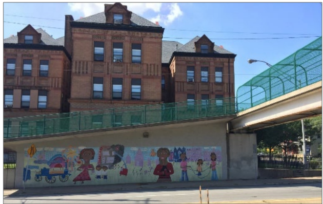
Figure 9 – Pedestrian bridge at Elmore and Beekman, with murals. Image Credit: Renaissance Planning
