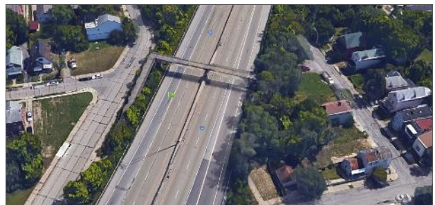
Figure 6 – The pedestrian bridge over I-74. Credit: Google Earth
