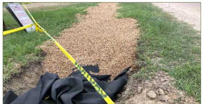
Figure 11 - Stormwater drainage being installed. Image credit: EPR
