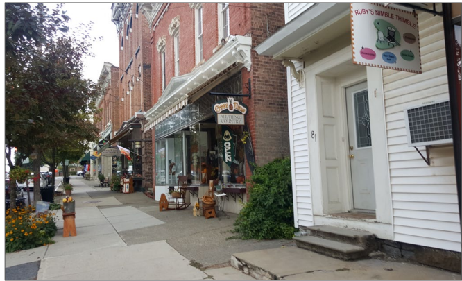
Figure 1 – View of Main Street shops in downtown Greenwich. Source: Renaissance Planning
