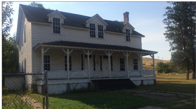
Figure 7 – Officer's barracks building, owned by National Park Service, southwestern end of Fort Lapwai. See map in Figure 6 for location (red outline). Image Credit: Jen Walker
