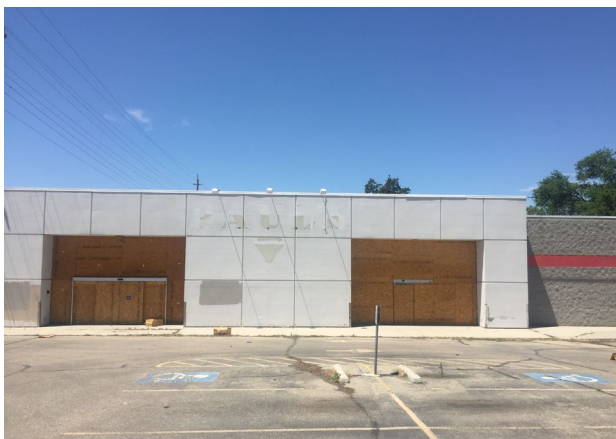
Figure 2 – The site of the former Paul's Market, closed since 2013. Image Credit: Renaissance Planning
